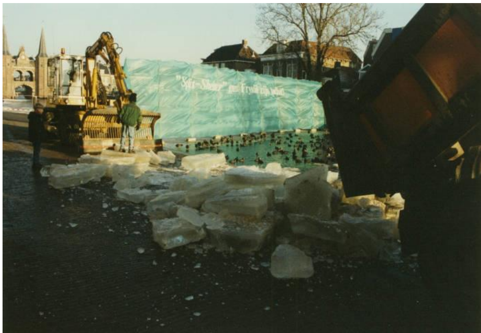
Figure 3: Conducting an ice transplantation in a ' wak ' near the old Waterpoort in Sneek in preparation for a possible fifteenth Elfstedentocht. The ice is delivered here by truck.
