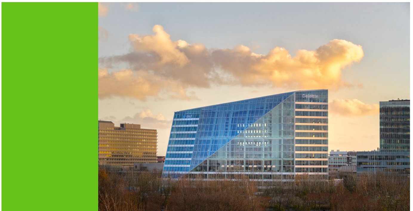
Deloitte Netherlands Office, 'The Edge,' named as one of the world's most sustainable offices in 2015.
