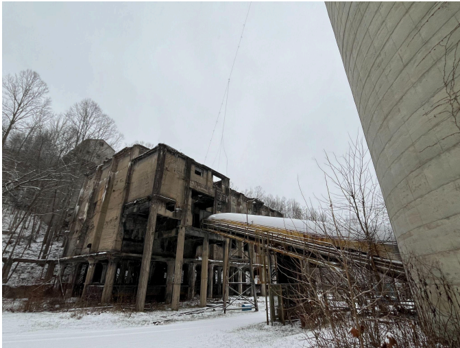
Figure 7: The old coal mine in the middle of the town
