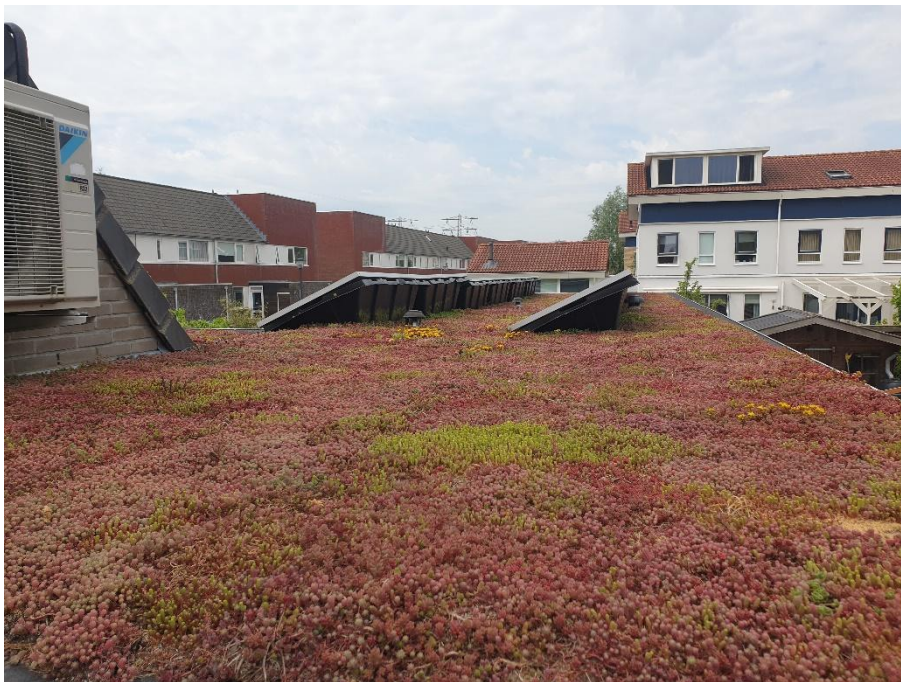
Figure 4.15 Extensive green roof in Leeuwarden (own photograph)
